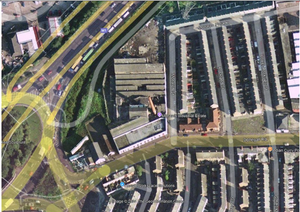
Monarch Laundry site prior to demolition
