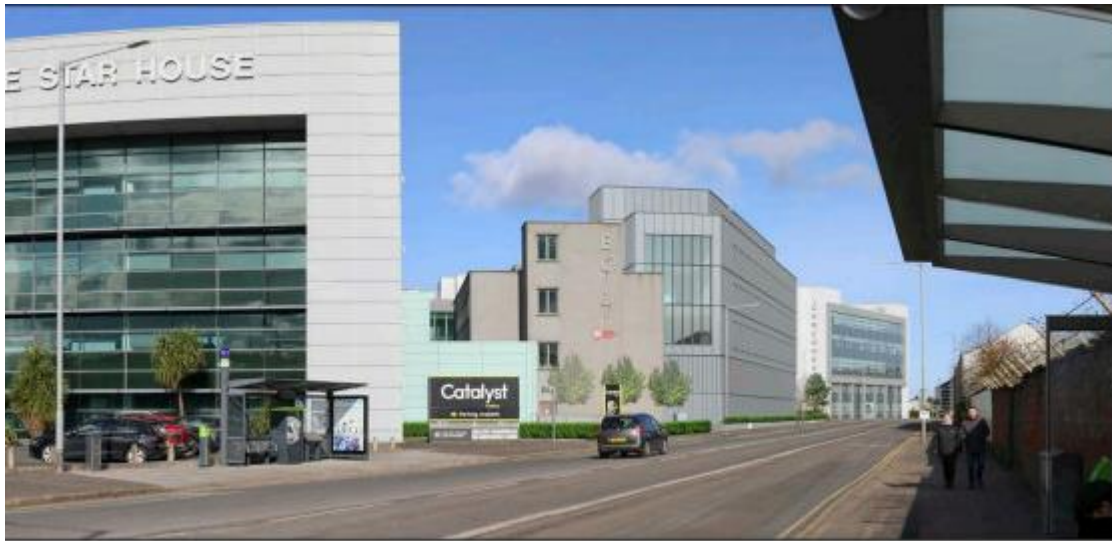
View from Queens Road (looking south):
